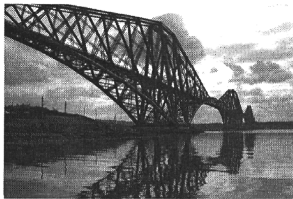
Fig. 14. The Forth Bridge
