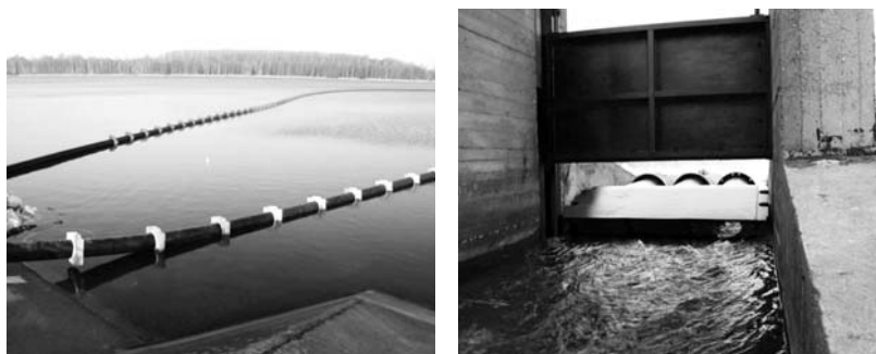
Fig. 2. Hypolimnion discharge channel with the Olszewski tubes
