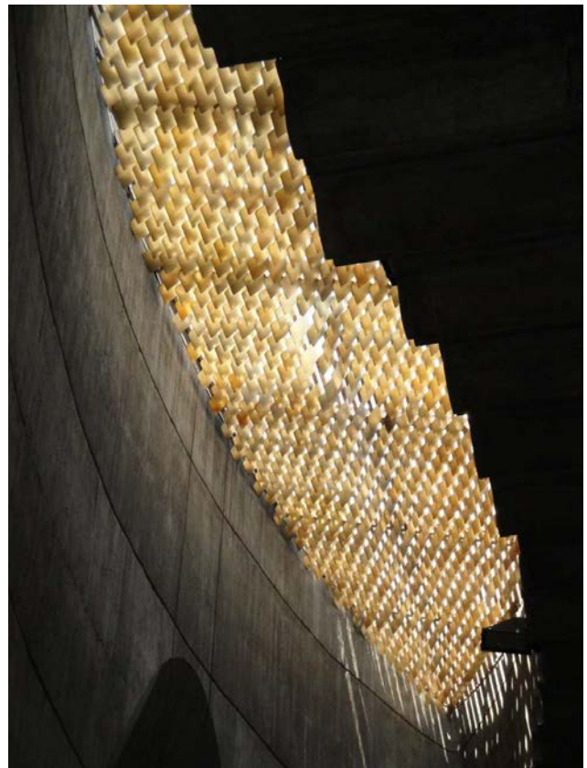
Fig. 5. Rooflight above the presbytery.
