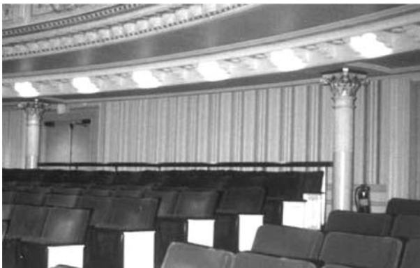
Fig. 2. Schroeder diffusers (QRDs) applied to the rear wall of Carnegie Hall to prevent echoes.
