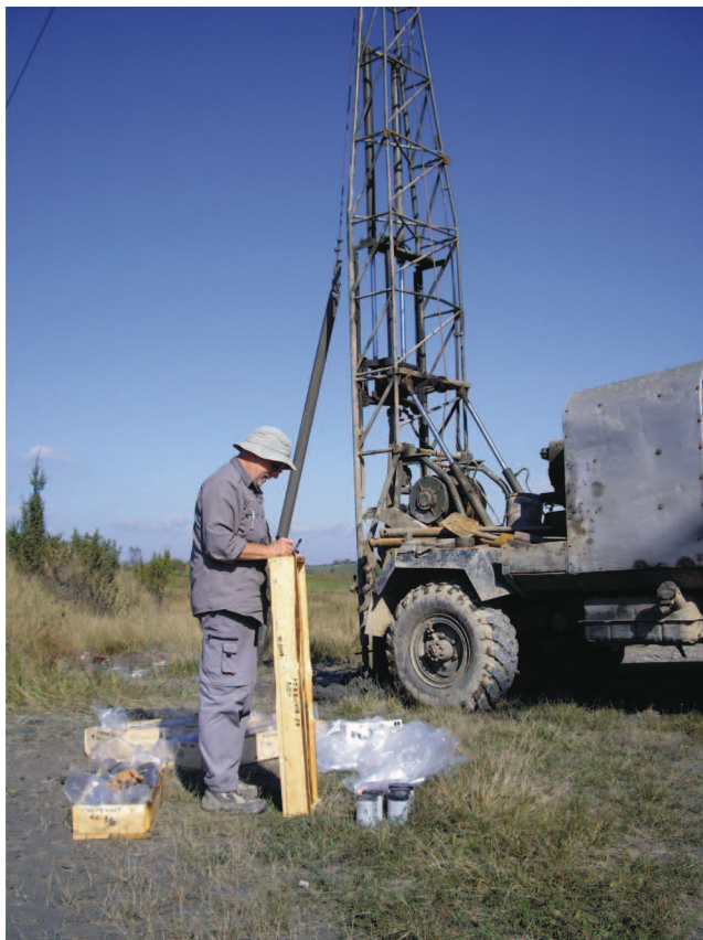
Fig. 10. The geological drillings by means of the UGB-50 vibratory probe (12 cm diameter) and core description by T. Sokolowski. Photo by R. Stachowicz-Rybka
