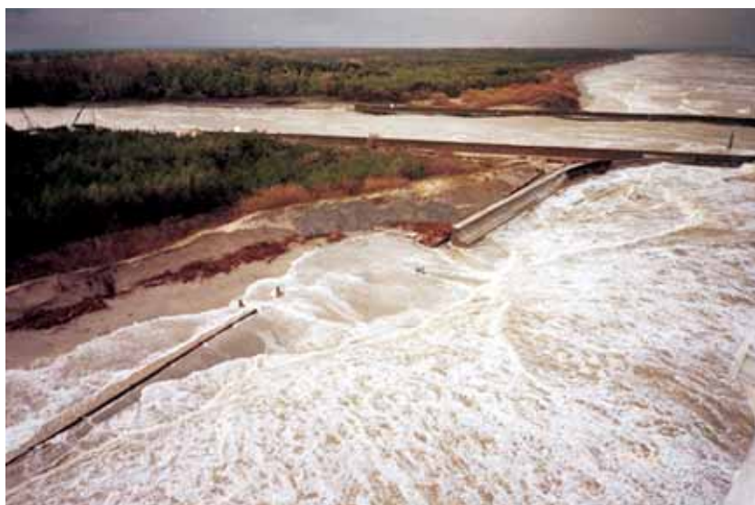
Fig. 8. Braking of Dziwnów Barrier (western Polish coast) during the storm in November 1995 (Photo. by P. Domaradzki)
