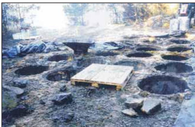
Fig. 3. Terrain of repository after excavation, before liquidation of stable construction
