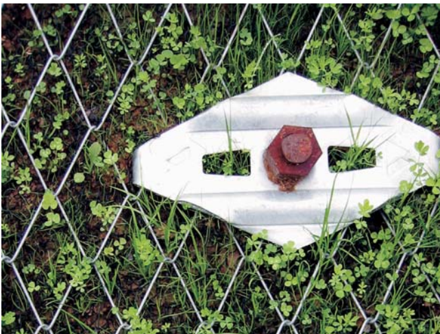
Fig. 6. High-tensile steel wire mesh TECCO
