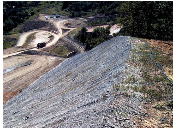
Fig. 8. After the mesh installation
