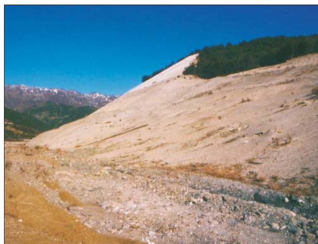
Fig. 4. Shotcrete facing at location D
