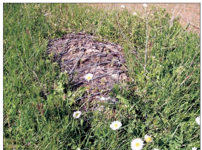
Fig. 10. A detail view of the mesh installation
