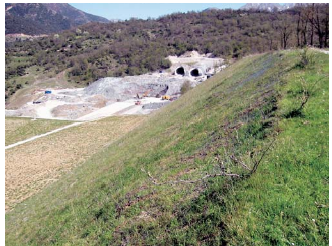
Fig. 9. After the mesh installation (one year later)
