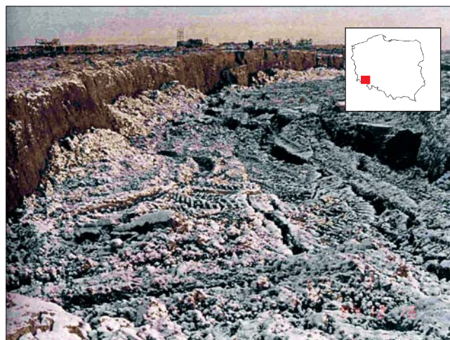
Fig. 2. Landslide on external embankments of Turów open-cast mine (6 mln m 3 )
