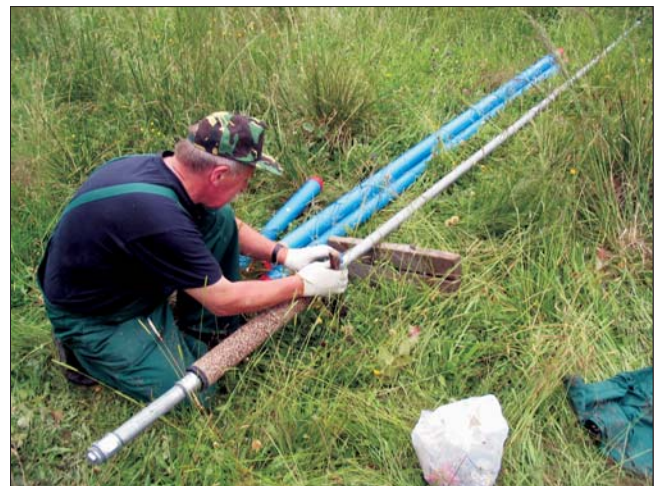
Fig. 15. Installation of Poltegor type standpipe piezometer
