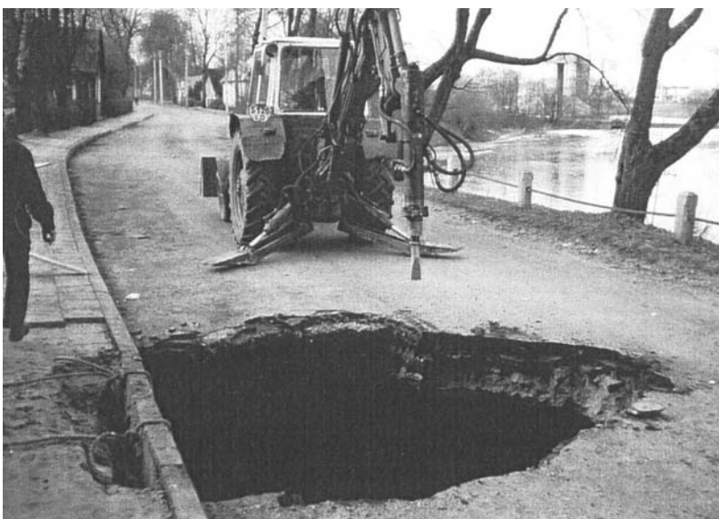
Fig. 2. The sinkhole formed in January 7th, 1999 in Pasvalys, the urban area most affected by karstic sinkholes in the North Lithuanian karstic area (photo by V. Mikulėnas)
