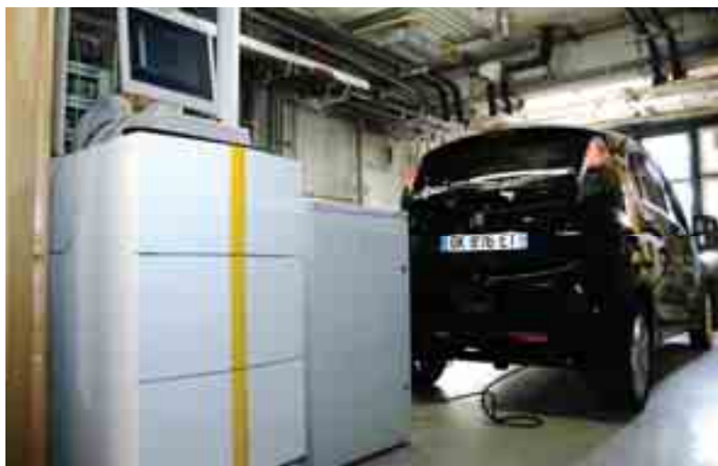
Fig. 2. An Electric Vehicle (right), charged from a stationary “early market” commercial SOFC power unit (middle). This SOFC also “transfers” the waste heat to the domestic water tank (left)
