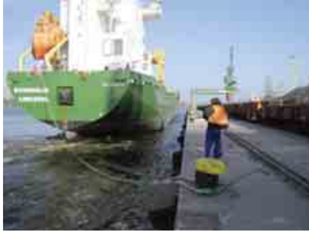
Fig. 1. The example of ship's berthing to Chorzowskie Quay in Port of Szczecin
