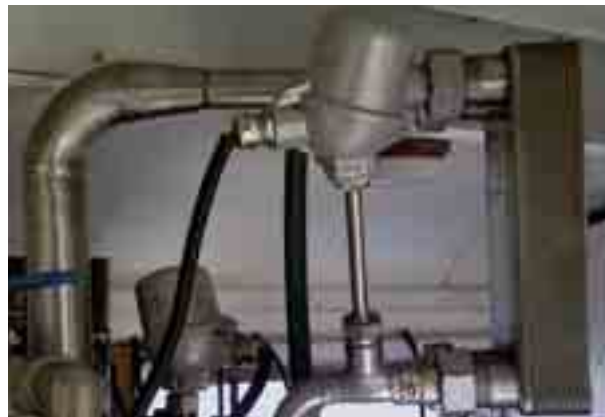
Fig. 6. A temperature sensor of the mixture temperature, alcohol condensate with a heat exchanger
