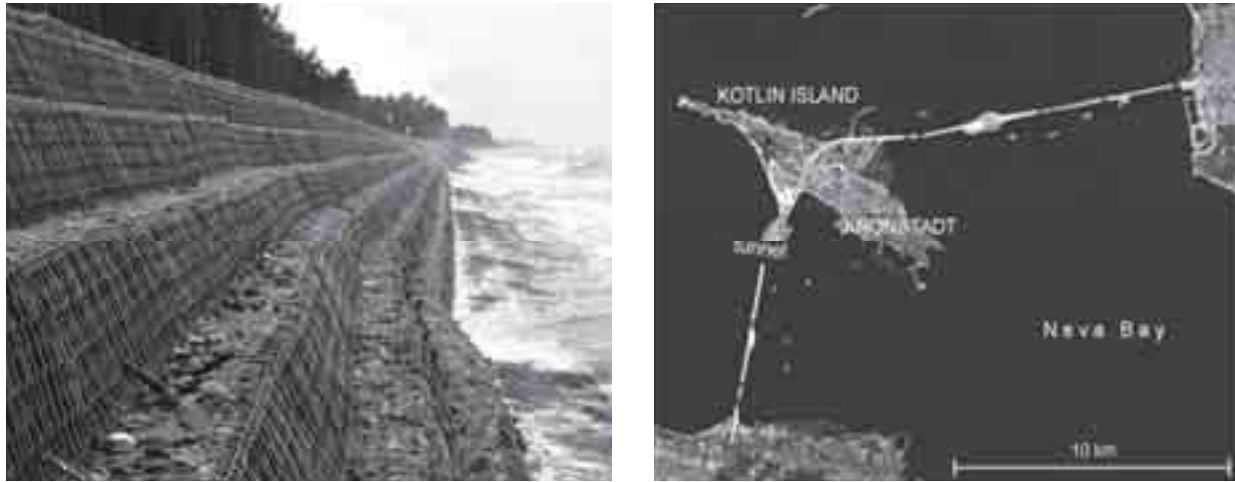
Fig. 4. Large scale coastal protection of the cliff-coast in Poland (left), the St. Petersburg (Russia) combined communication connection and flood barrier (right)
