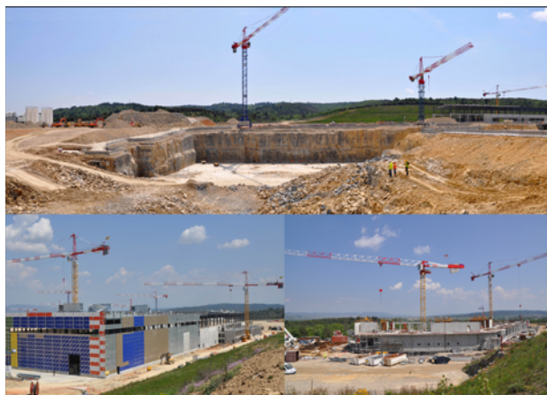
Fig. 1. Construction progress in May 2011 on the ITER site.
