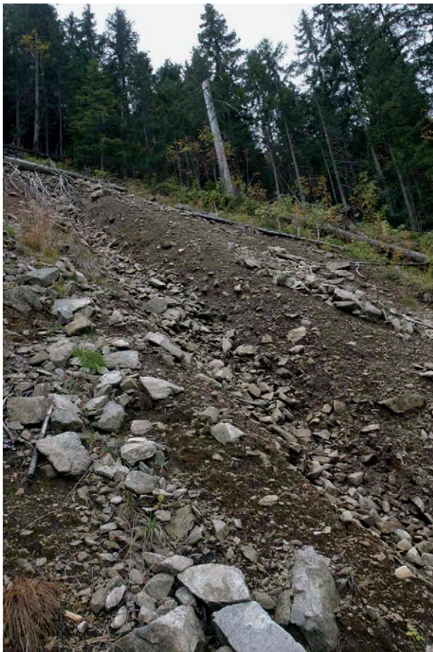
Fig. 1. Landslide located on the slopes of Czuba Roztocka in Roztoka Valley
