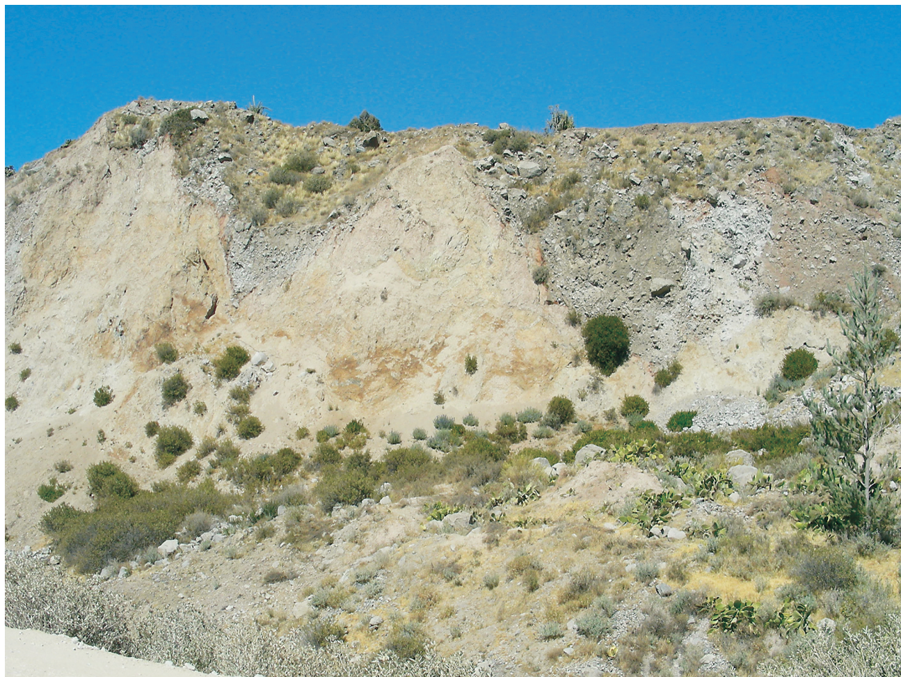
Ryc. 9. Młode szczeliny w koluwiach osuwiska w Maca Fig. 9. Young fractures in colluvium of the landslide at Maca
