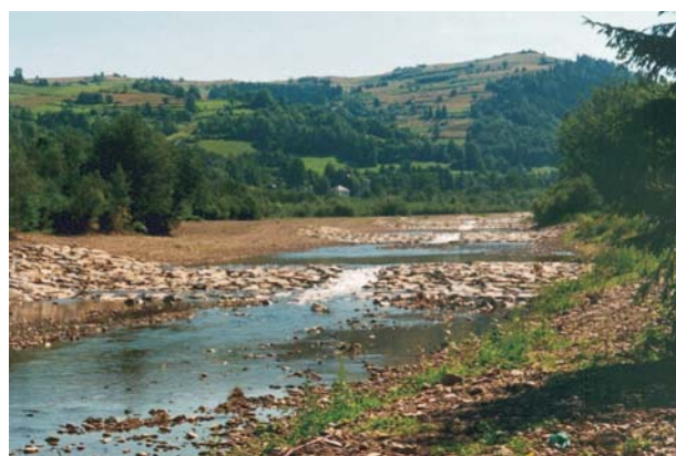
Fig. 5. The rapid hydraulic structure in the Porębianka River in Podobin
