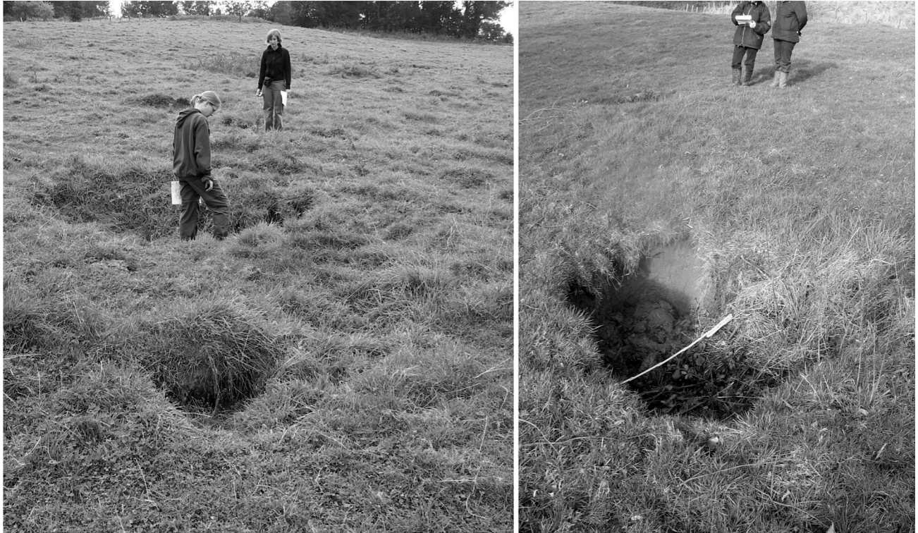
Fig. 1. Collapsed pipes in Kluisbergen (left) and Ronse (right), Belgium
