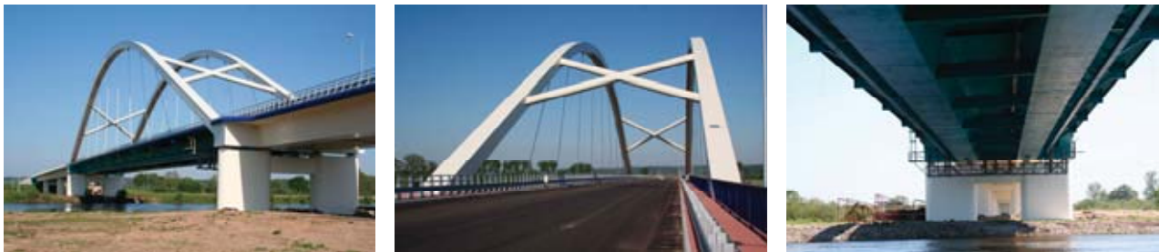
Fig. 7. Construction of the arch stayed span of the bridge in Gorzów Wielkopolski
