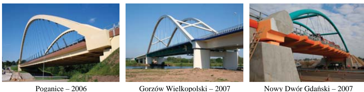
Fig. 2. Pictorial view of the analyzed overpasses
