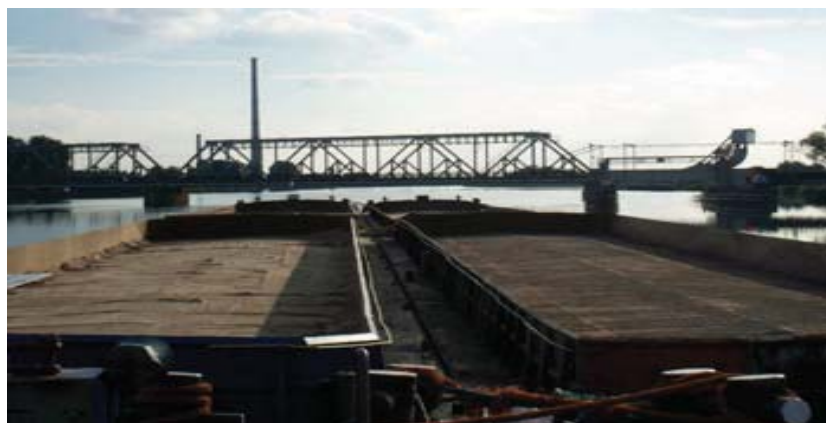
Fig. 2. The railway bridge (Podjuchy- Szczecin)
