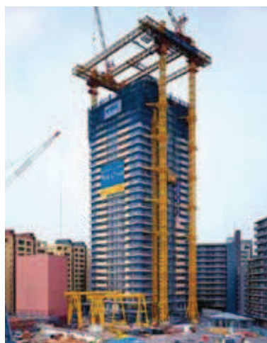
Rys. 12. Shimizu Smart system
