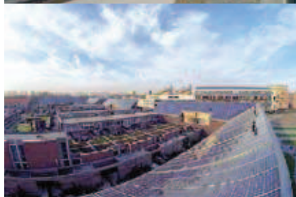
Holandia, Amsterdam Nieuw – Sloten BIPV houses
