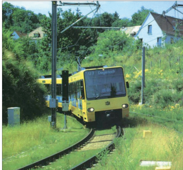
Fig. 1. City railway Stuttgart, Germany. Example of a greened up geogrid reinforced soil structure (1990).
