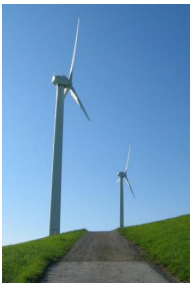
Rys. 1. Badane turbiny wiatrowe Tacke Tw 600 Fig. 1. Tested wind turbines Tacke Tw 600
