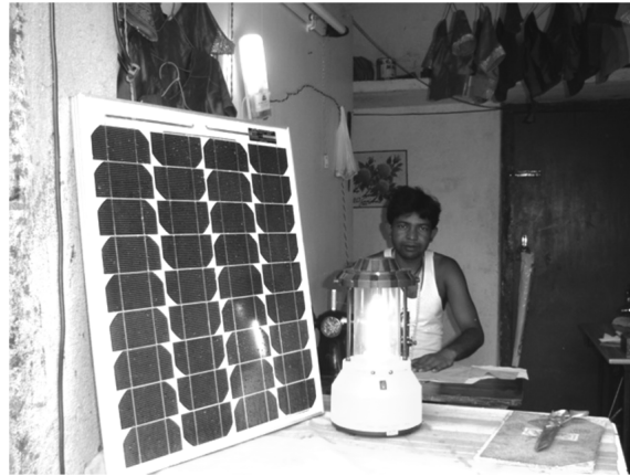
Figure 11. Power saving observation of SPC installed at a tailoring house located in rural sector of Jamshedpur city.
