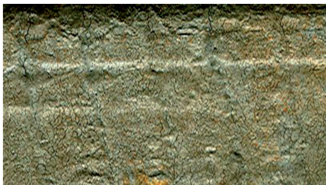
Fig. 2. Cracks on the surface of an S355J2-NbTi steel continuous cast billet
