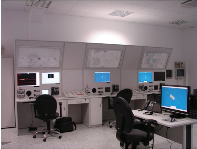
Fig. 2. Radar position: PAR (on the left) and APP (on the right), in the middle APP assistant's position (phot. T. Compa)
