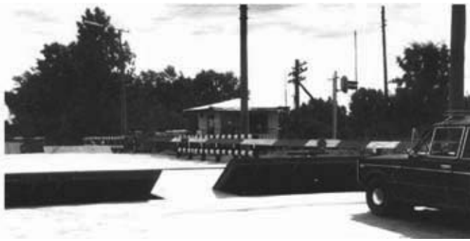
Fig.3. Mechanical ramps obstructing the entrance to a level crossing (Russia)
