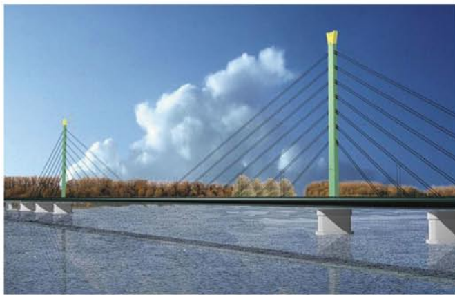
Rys. 4. Nowo zbudowany most podwieszany nad Wisłą [2] Fig. 4 Newly constructed cable-stayed bridge crossing Vistula River [2]
