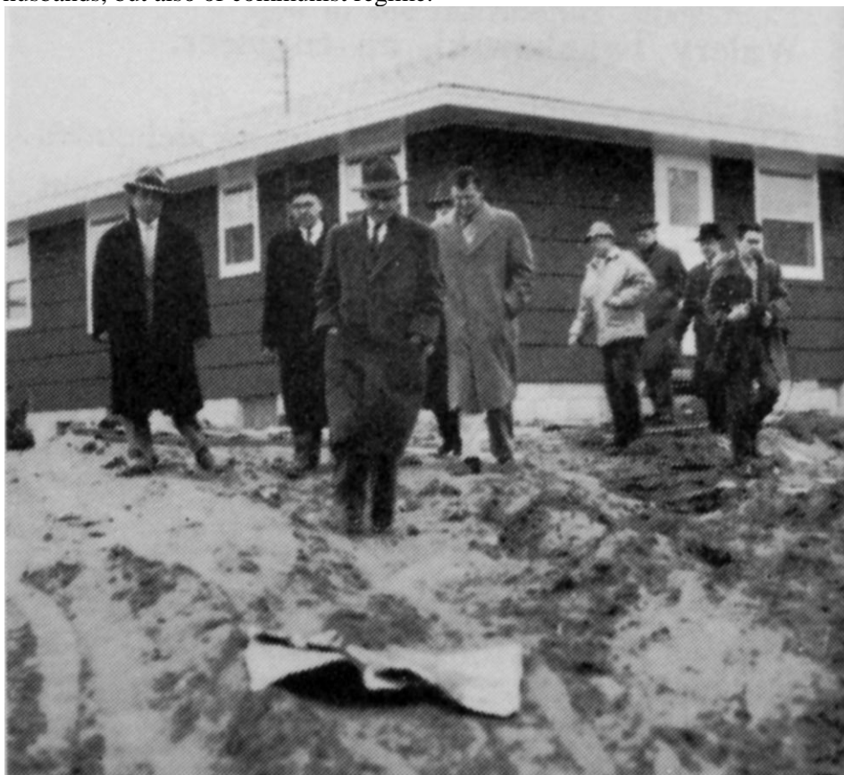
Fig. 4. On construction site in Minneapolis.
