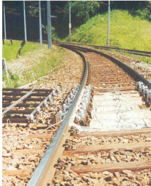
Fig. 5. The measurement site in the ballasted track (see the rail corrugations!)
