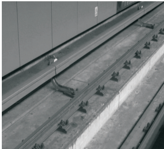
Fig. 5. The railroad in the tunnel of the underground train
