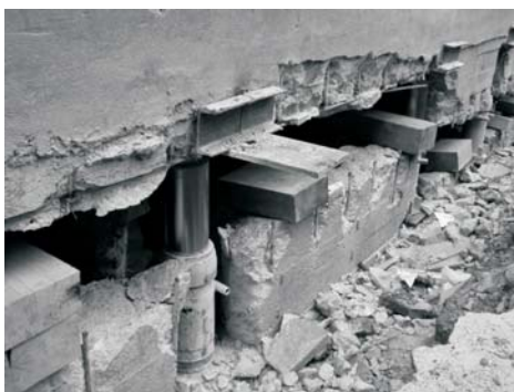
Fig. 5.1. Rectification with the help of boosters
