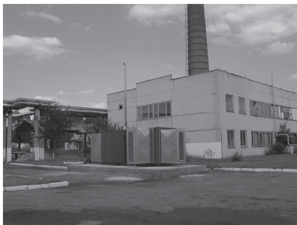
Fig. 5. Overview of diesel power station, working on rapeseed oil in Khoyniki.
