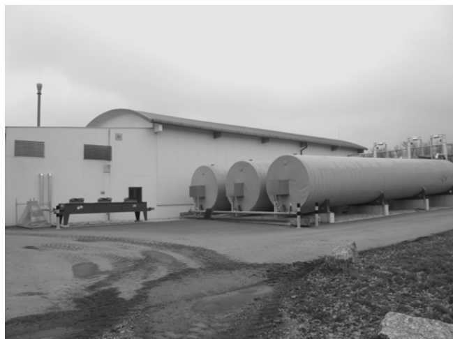
Photo 2. A view of steel tube fermenters 8 (right part of photo) – BGS Amstetten (Austria) – photo by authors
