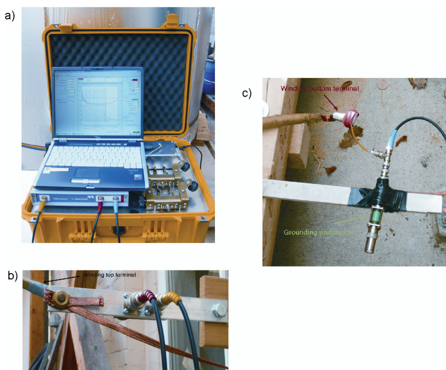
Fig. 4. The test setup: a) Bode 100, PC, and cable connection, b) Cable connections at the winding top terminal, and c) Grounding resistance and cable connection at the winding bottom terminal
