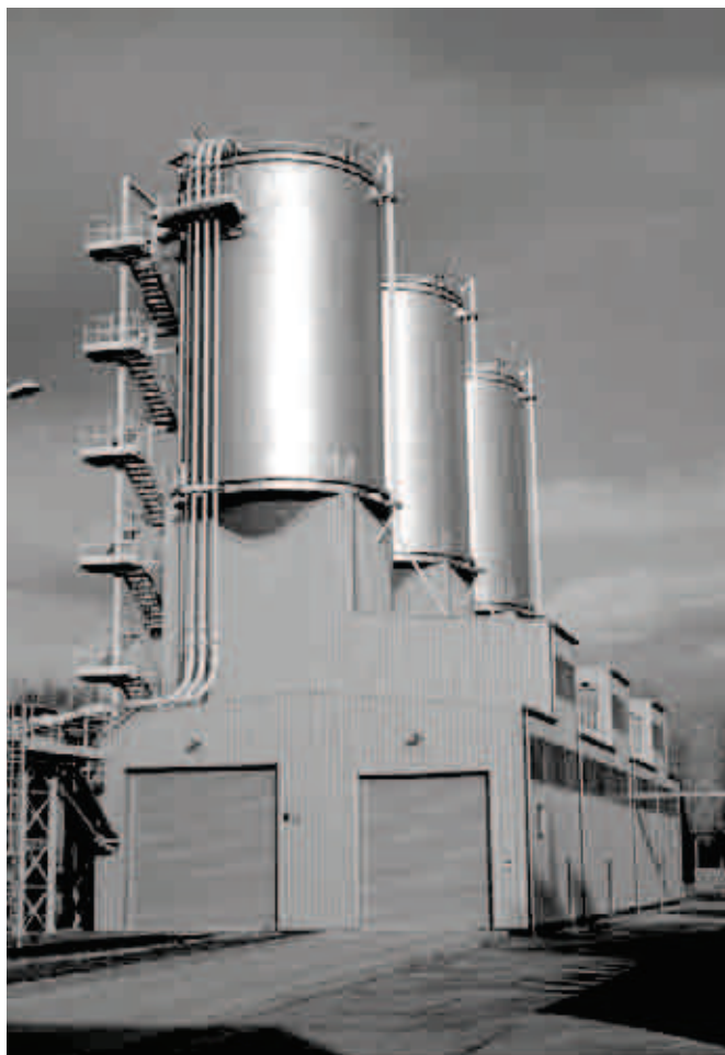
Pic. 3. Installation of dry ash collection
