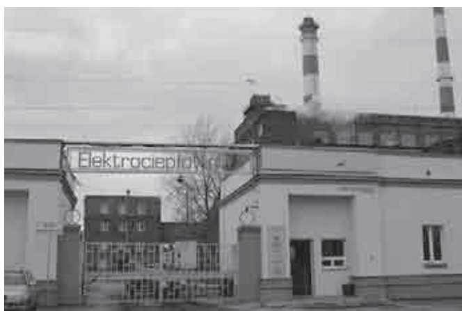
Fig. 1. Combined Heat and Power Plant
