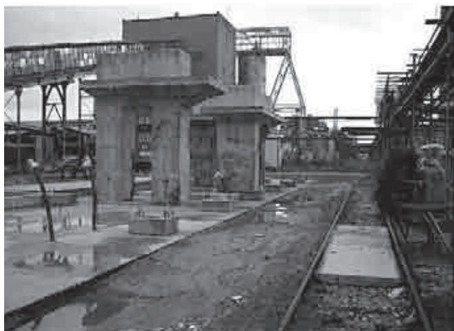
Photo 4. Preparation works regarding territorial development for the main installation
