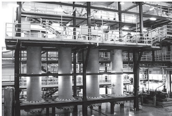
Fig. 4. View of extractors for hop extraction
