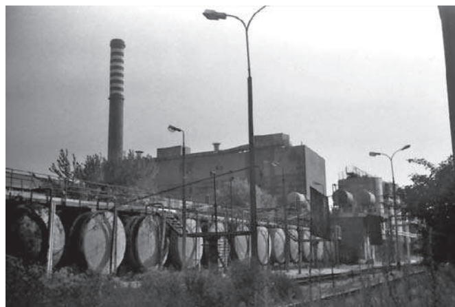
View of the sulphuric acid storage tanks (12 horizontal tanks, capacity 100 m 3 each, 2 head tanks on the building, further away vertical tanks for soda lye), Wiskoza 2 plant building and stack of the Central Ventilation Station No. 1 (1980)
