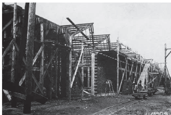
Construction work at a building of one of the first fibre plants (March 1909)
