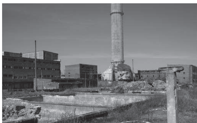
Abandoned factory buildings, in the foreground water pits where carbon disulphide storage tanks were once installed (these tanks were placed in water pits for safety reasons) (1999)
