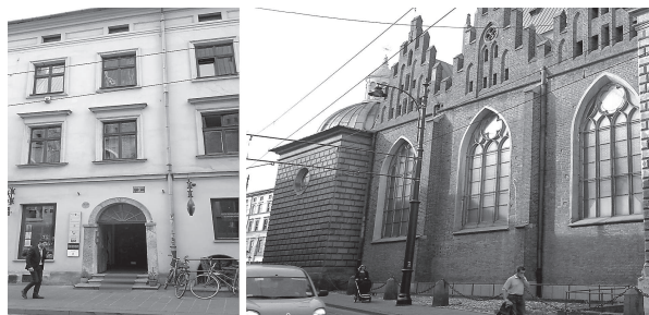
Fig. 8. On the left: No. 3 Dominikańska street. On the right: the Holy Trinity Church from the direction of Dominikańska street. From left to right, the church's chapels are: Lubomirski Family Chapel, St. Thomas' Chapel, the Saviour's Chapel, St. Joseph's Chapel, St. Dominic's Chapel (chapel of the Myszkowski family), and the Chapel of the Rosary
