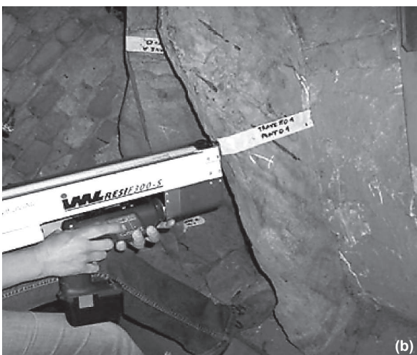
Fig. 8. Sampling of the wooden structure for identification: from the joist (a); from the rib (b); and from the reed mat (c)
