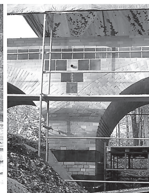
Fig. 16. Surface of bridge after cleaning
