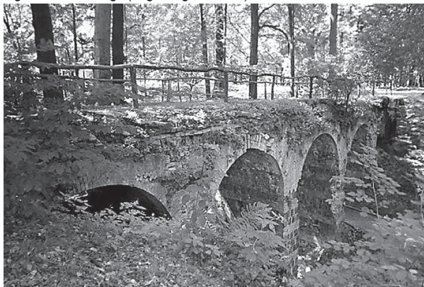
Fig. 10. Arcade Bridge (1990s)
