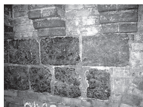
Fig. 17. Arcade Bridge – built-in original structural elements
