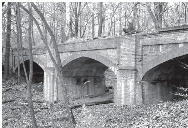
Fig. 2. Royal bridge (before 1999)
