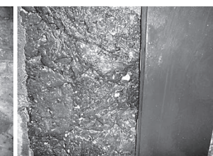
Fig. 18. Arcade Bridge – original and new elements made of glass slag
