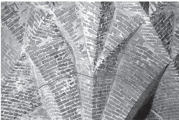
Fig. 8. The exposed masonry texture of the analyzed vaults shows the continuity of the courses over large portions, across the discontinuities of the vault surfaces (cf. also Figure 3). This is not conform with modern masonry rules and contradicts the current descriptions models, but in the experiments turned out to be very practical (D. Wendland)
