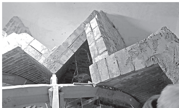
Fig. 13. Also in the higher portions the continuity over the whole squinch can easily be maintained. Over the transversal cap, the courses are seamed (D. Wendland)
