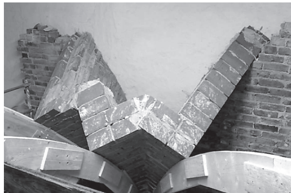
Fig. 11, 12. Details of the experimental reconstruction. The vault masonry is executed without formwork on single centering arches supporting the groins. The thickness of the shell is according to the archaeological evidence. The peculiar masonry texture with the continuity of the courses over the inward folds, as observed on the original vault, turned out to be practical (D. Wendland)
