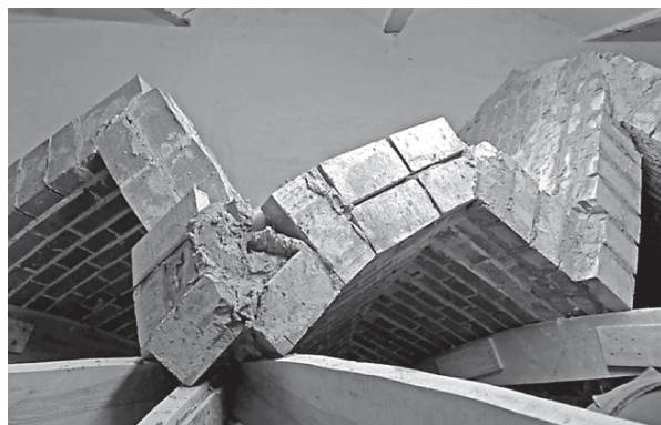
Fig. 14. At the intersection points in the groins, the direction of the masonry courses change. Nevertheless, the continuity of the texture is maintained (D. Wendland)
