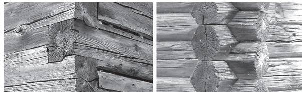
Fig. 7-8. Short corner and long corner of old Finnish log buildings
