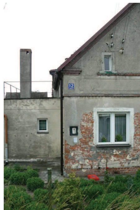
Rys. 6. Monitorowany stary budynek Fig. 6. Monitored old building
