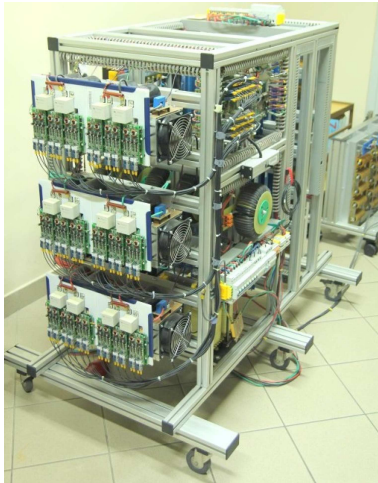
Fig. 14. A laboratory model of the power conditioning system based on a five-level cascaded converter and supercapacitor energy storage (height 1 m, mass 300 kg)
