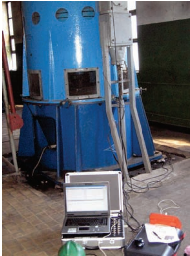
Fig.1. Electrical motor of mixed flow pump
