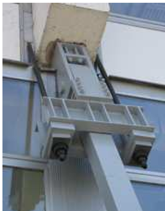
Fig. 9. The lower joint of the by-pass construction.
