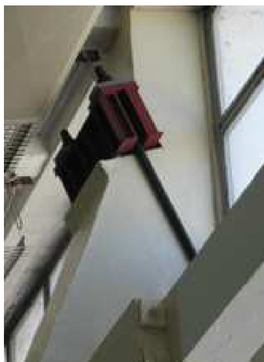
Fig. 10. The upper joint of the by-pass construction.
