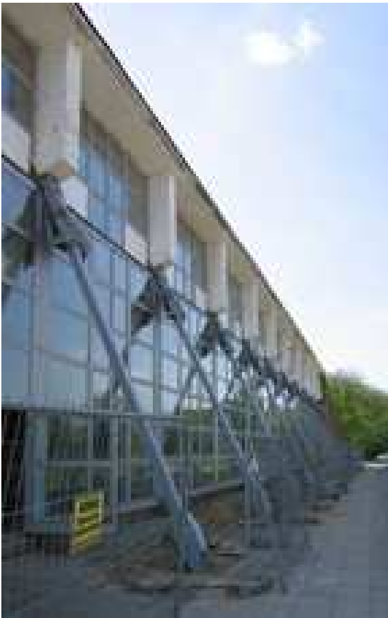
Fig. 11. The restored column line.
