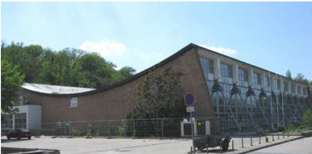
Fig. 1. The indoor swimming pool.
